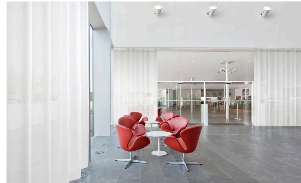
'Liquid' translucent acoustical curtains are used in front of glazing throughout the atrium.
